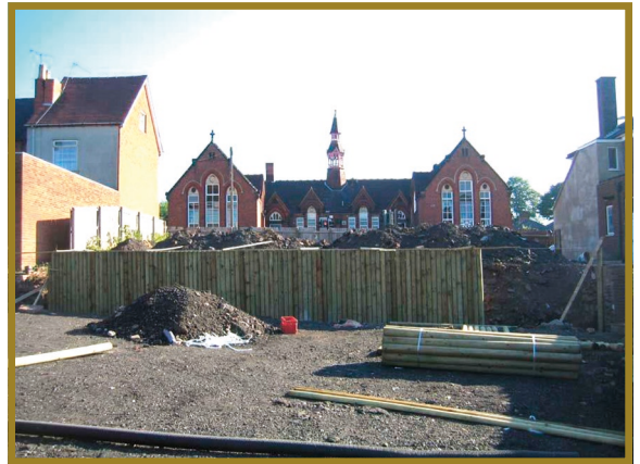
Work in progress: site cleared and ground work underway.
