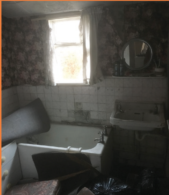
Bathroom before renovation.
