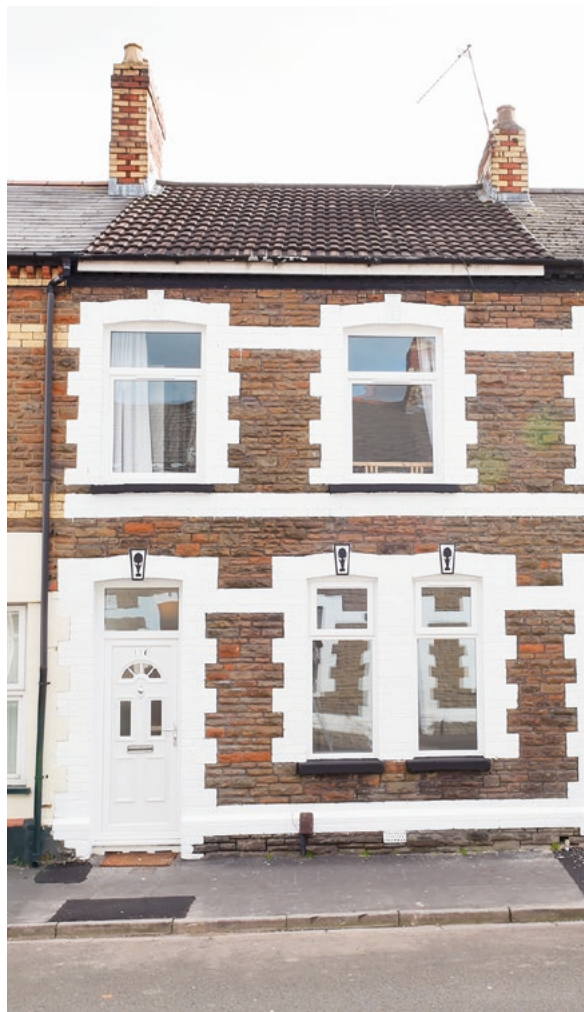
Carlisle Street following renovation.
