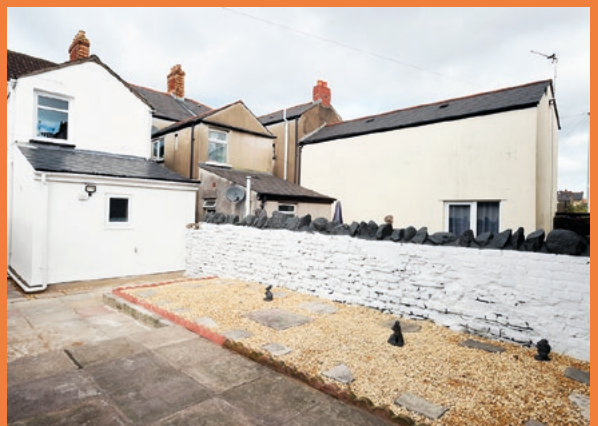
Garden after renovation.
