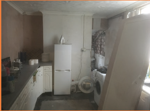
Kitchen before renovation.
