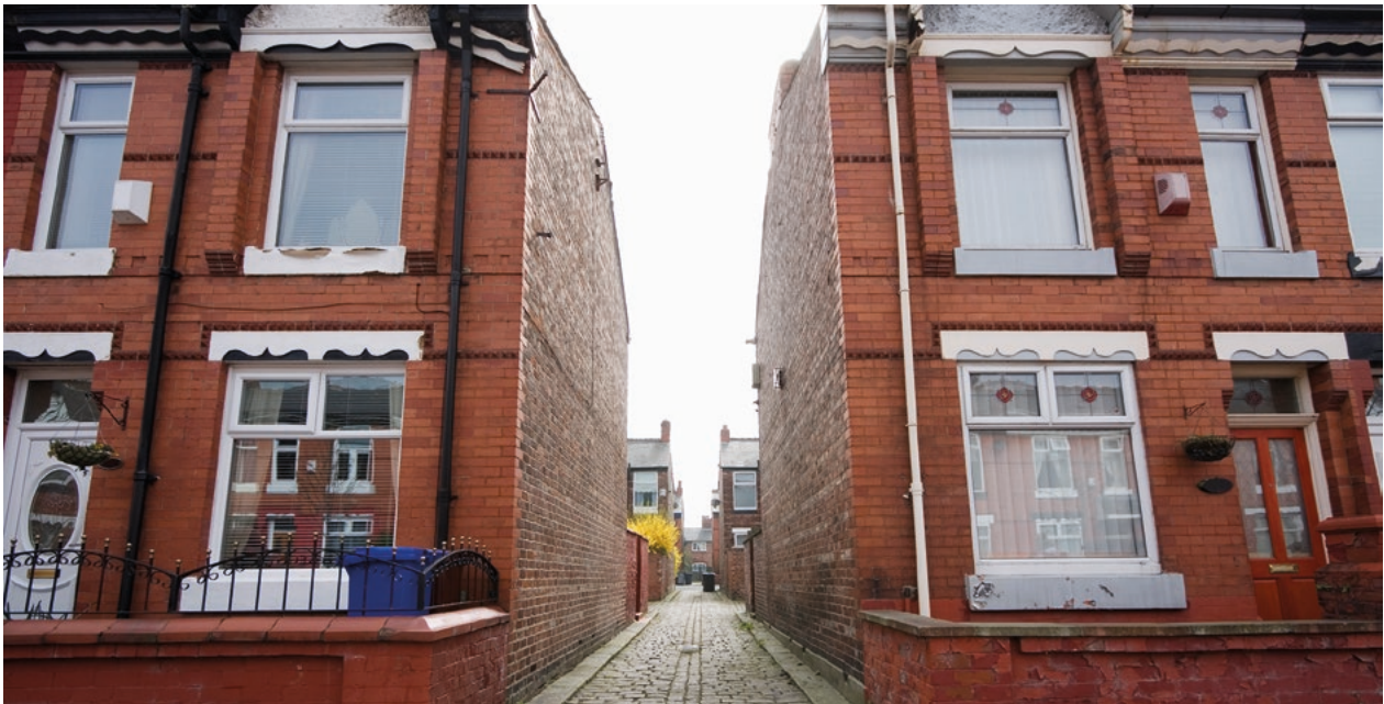
The economic pull of Manchester continues to be a major factor in the strength of the North West property market
