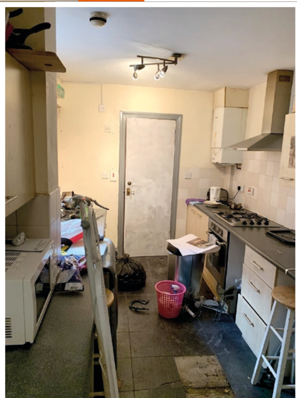
Below: kitchen before
