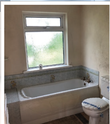
Right: bathroom before refurb
