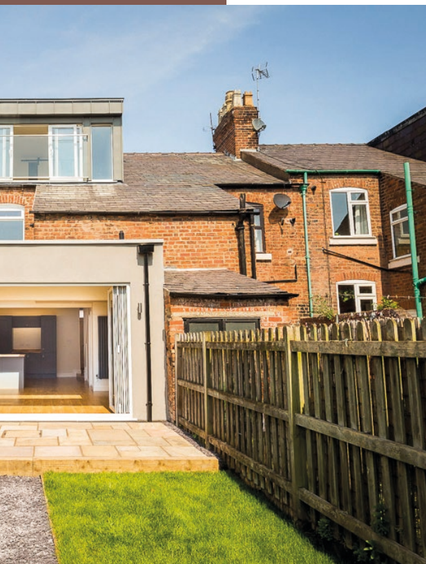
Above: the extension and renovated kitchen
