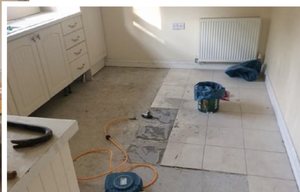
Above: removing damaged tiles from the kitchen floor
