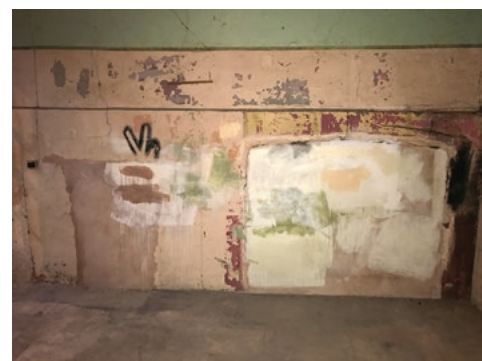
Below: bedroom before renovation
