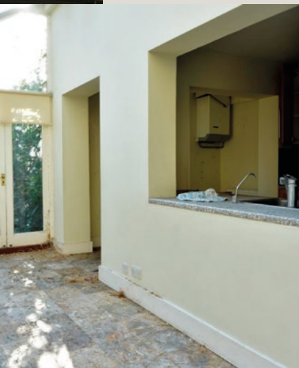
Below: dining area before refurbishment
