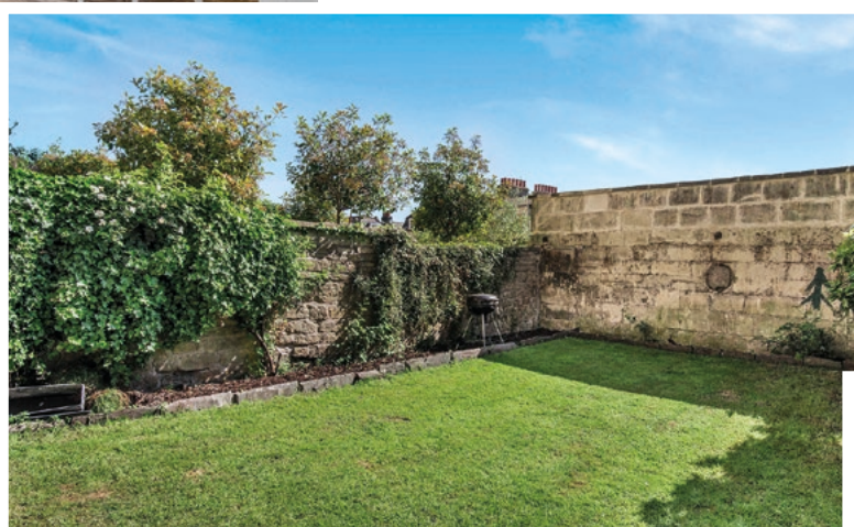
Above: garden after renovation
