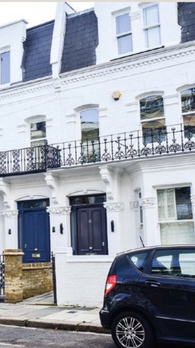
Front after refurbishment
