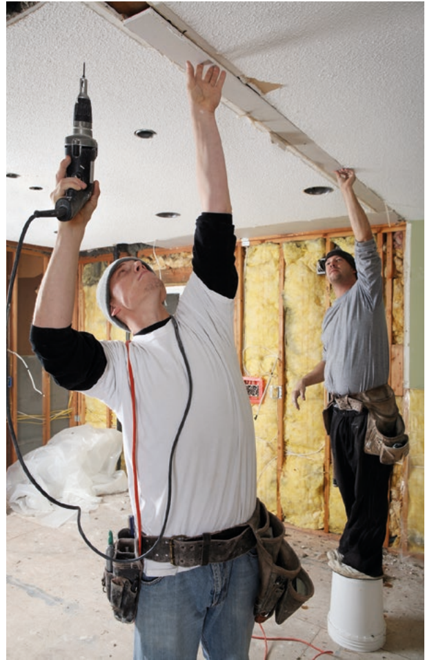
Retrofitting home insulation
