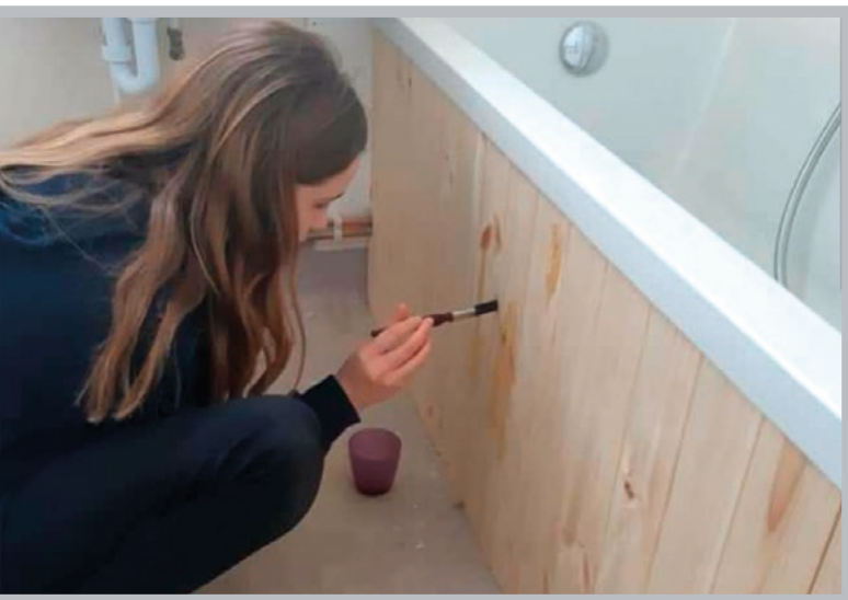
Above and left: Chelle and Mark's children helping out with renovation
