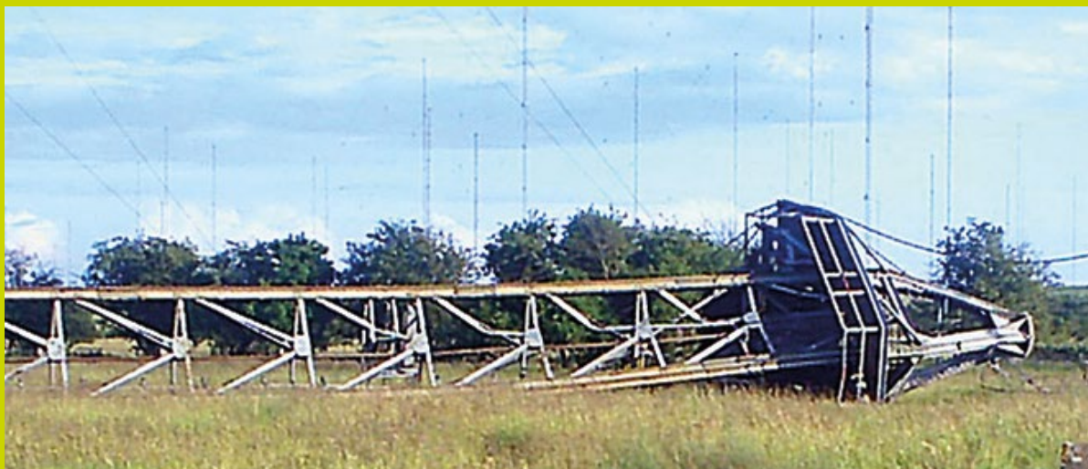
A fallen mast at the site of the former Rugby Radio Station, soon to be developed as a new village.
