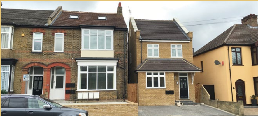
The completed properties.
