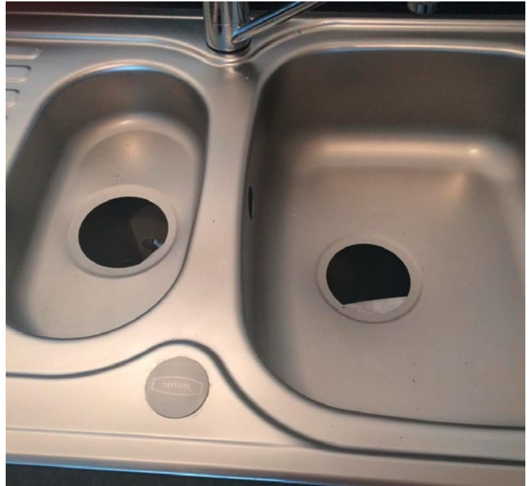
Make sure taps work efficiently, and ensure the water pressure is good.
