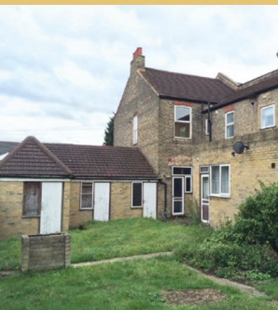
Renovating the existing house and building another on the same site.
