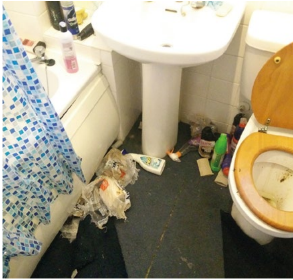
The bathroom needed completely re-installing: left – before and right – after the work.
