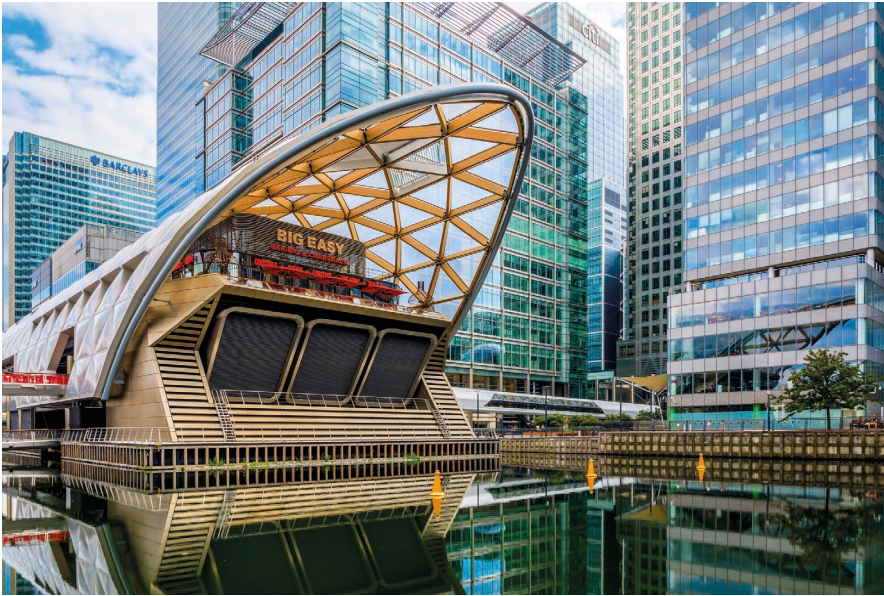
Crossrail station at Canary Wharf.
