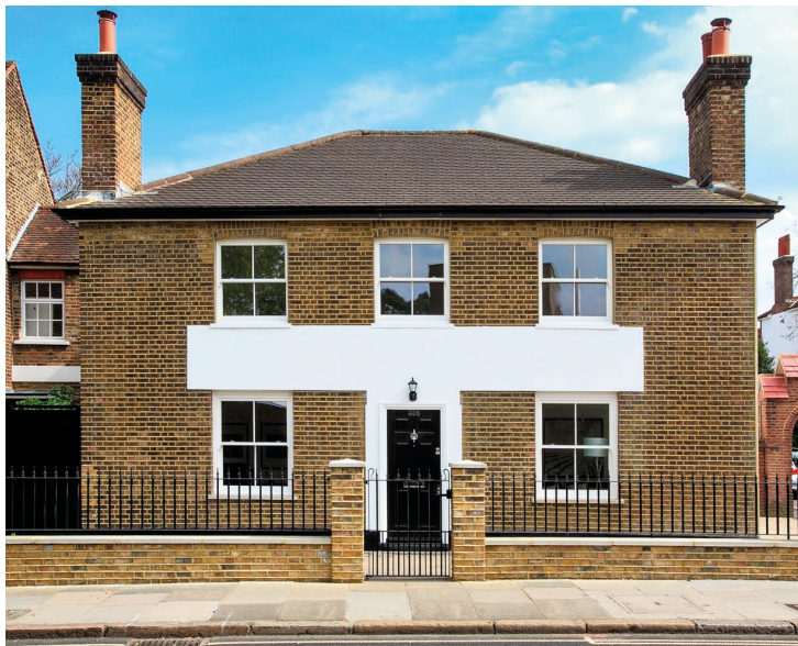
David Barker's refurbished Kew house.
