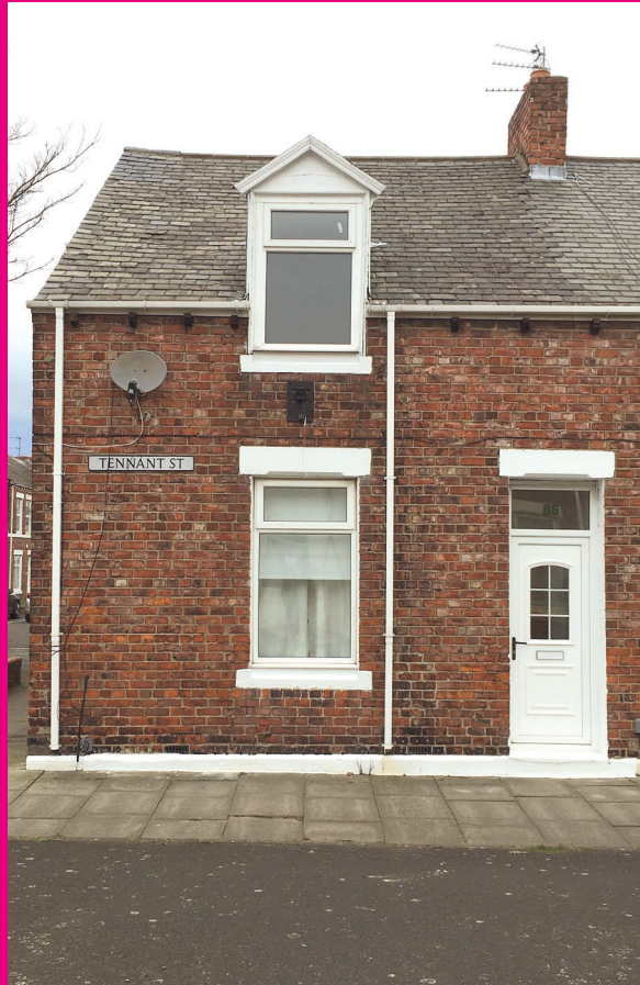
Tennant Street refurbished exterior.
