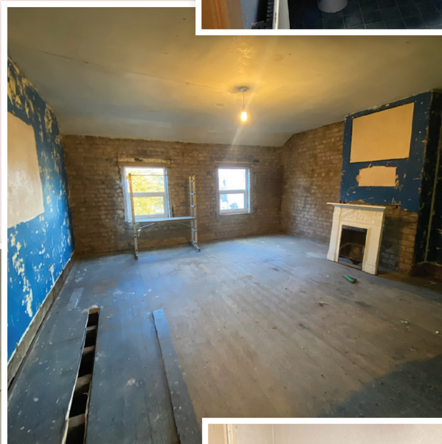
Their latest project was a full back-to-brick conversion
